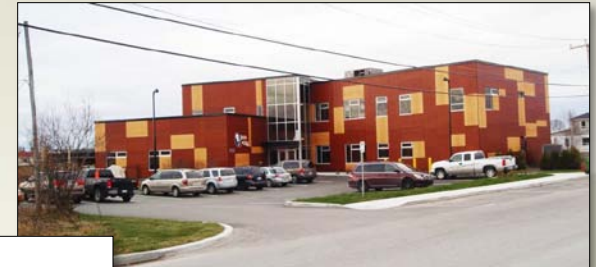
Day Care Facility
