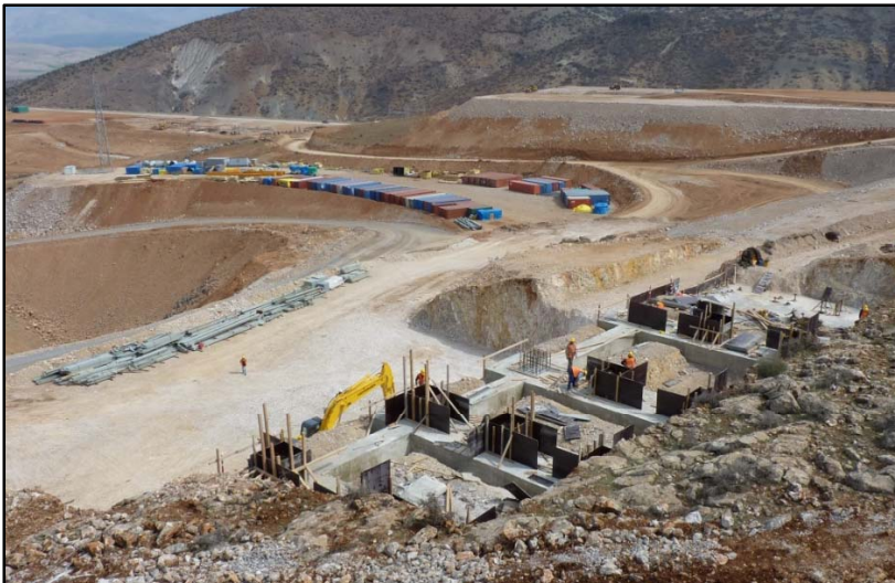
Secondary Crushing Plant & Bin Foundations – end of March '10
