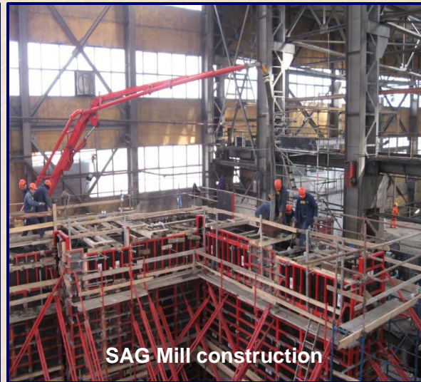
Construction of tank ring beams in flotation area of the existing mill
