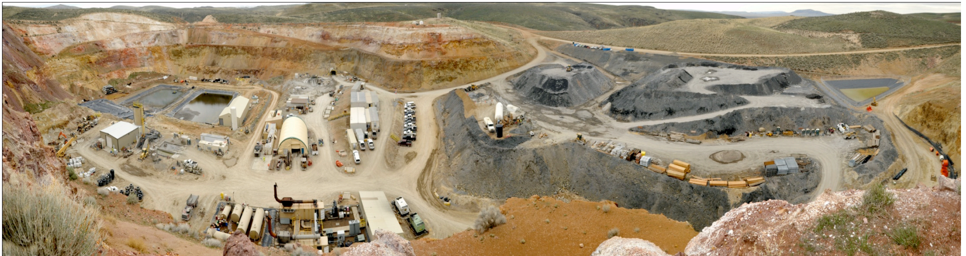
Hollister Project infrastructure constructed in previously mined open pits
