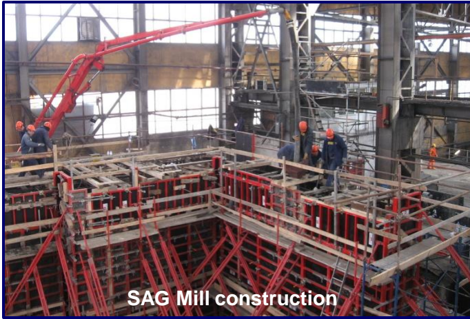
Early stage construction
