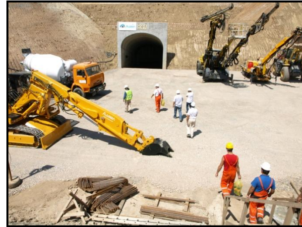
Vyara Portal Construction Q3 2010
