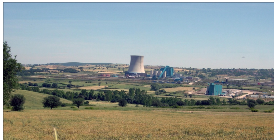
Electrical generating station in nearby Çan
