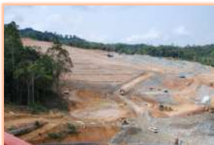
*Tailings Dam Earth Works
