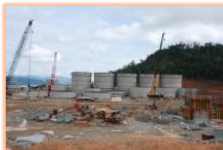
*Tanks in CIL area under construction
