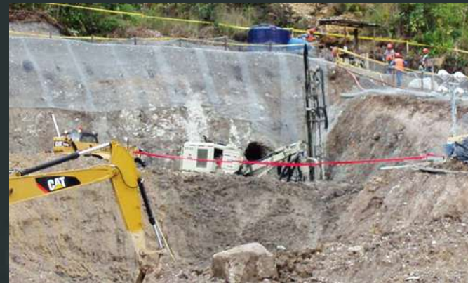
PORTAL HIGH WALL CONSTRUCTION
