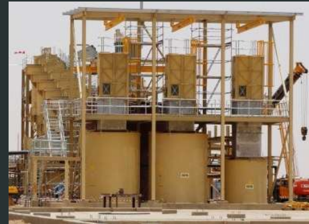
NEW ADR PLANT 74% COMPLETE
