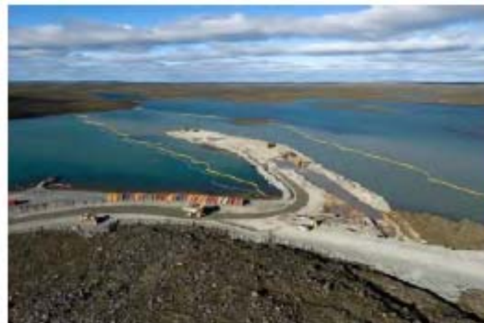
Cofferdam construction at Meadowbank Gold project, Nunavut
