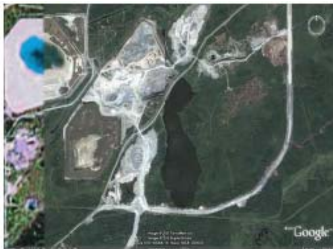
Cofferdam at Pamour Mine, Ontario
