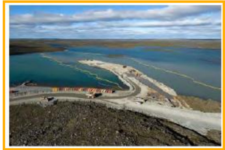
Cofferdam construction at Meadowbank Gold project, Nunavut
