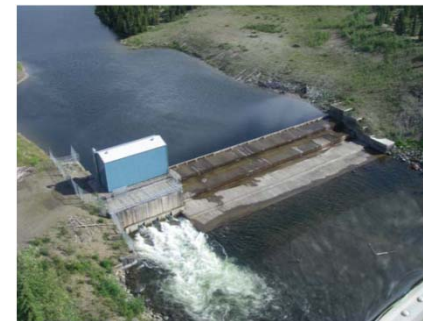
Mayo B facility
