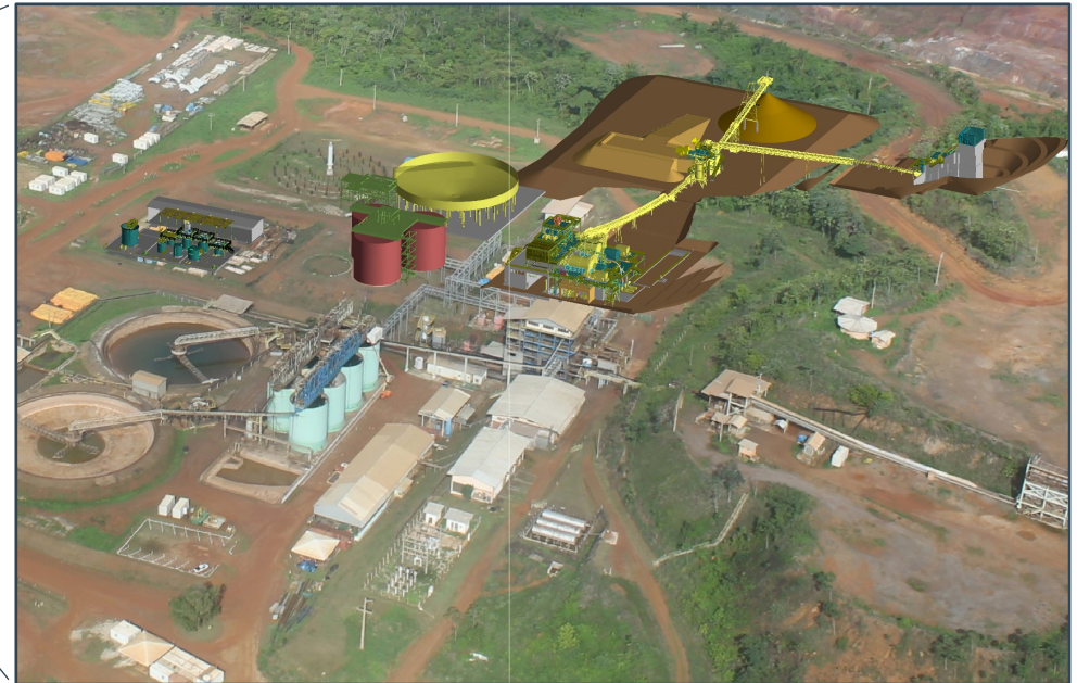
Aurizona Mine – Existing Infrastructure and Planned New Front End
