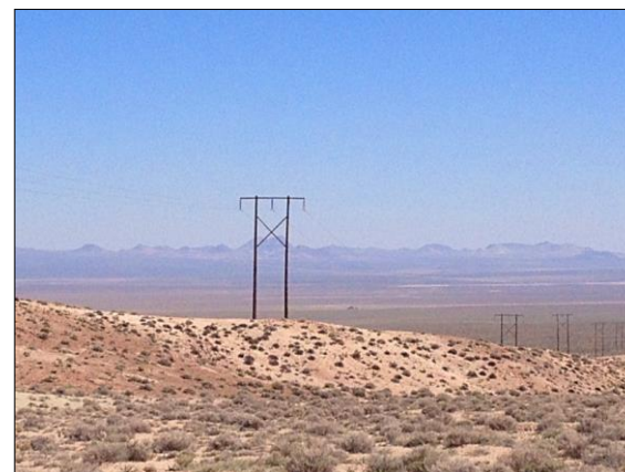
120 KV power transmission line passes through the property.
