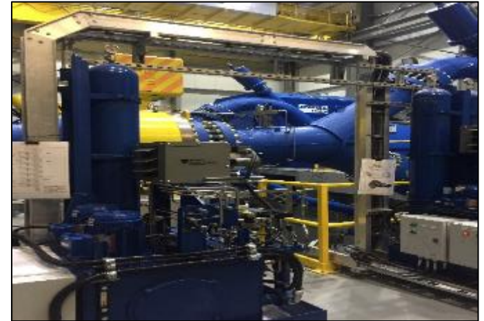
Regional's 31 MW Power Plant
