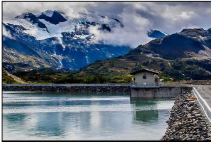
Long Lake Hydro Dam
