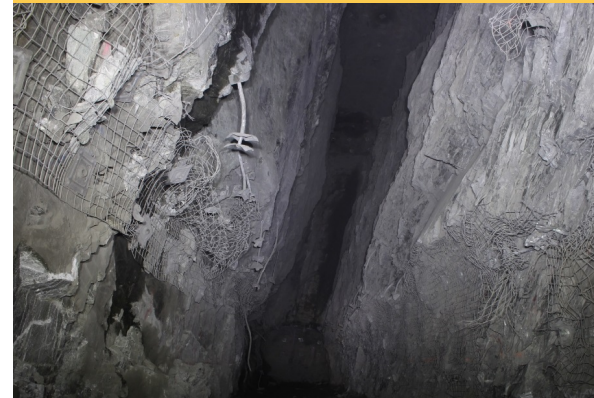
Stoping conditions at Beresford South
